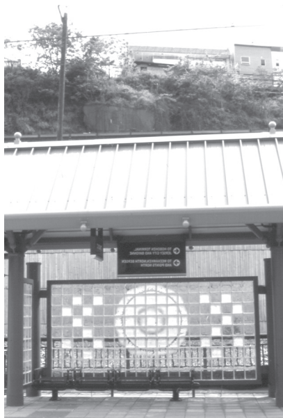
Second Street Station, Bergen–Hudson Light Rail, NJ Transit, Hoboken, 2004.
